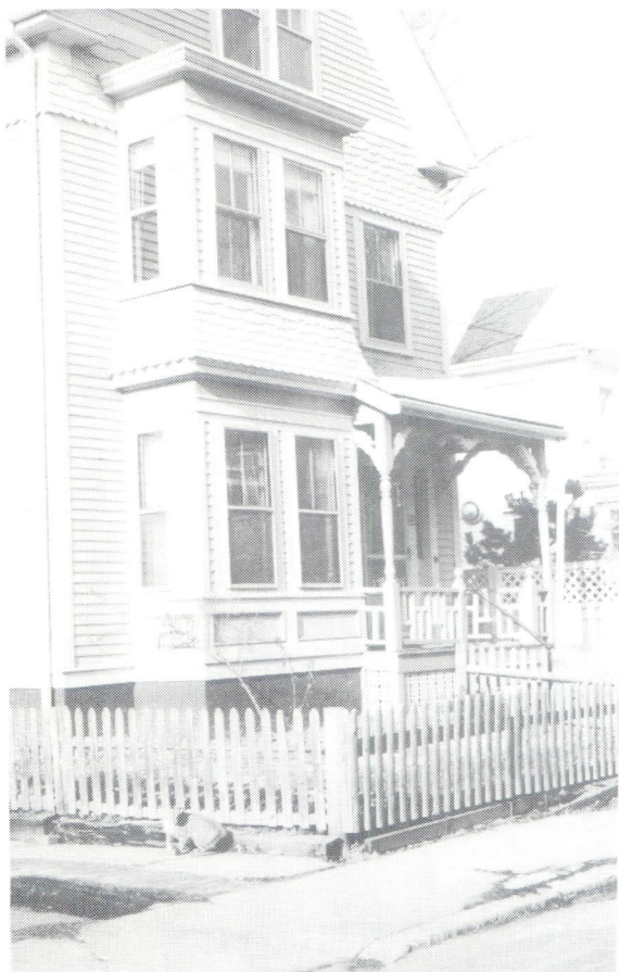
F5. Patterned shingled house, with cat (cat's name not necessary!)
