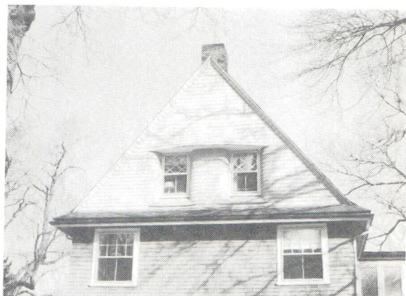
F17. Curving window hood in the gable
