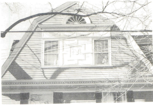
E15. Festooned panels with attic fan in gambrel gable
