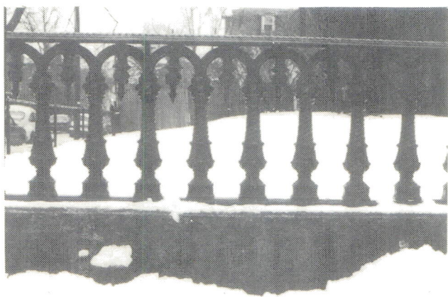
E6. Decorative iron work
