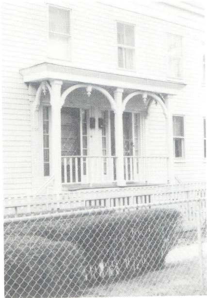
C12. Doubled-arched, double doorway
