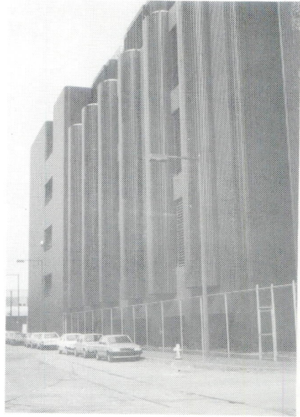
C5. Modern "silos"
