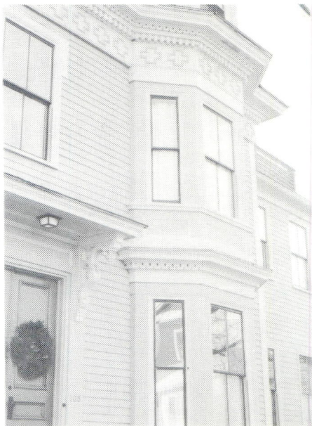
D5. Striking cornice detail
