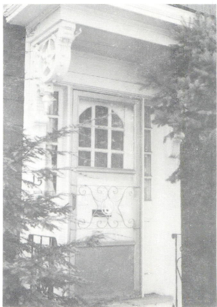
D19. Hefty entrance supports
