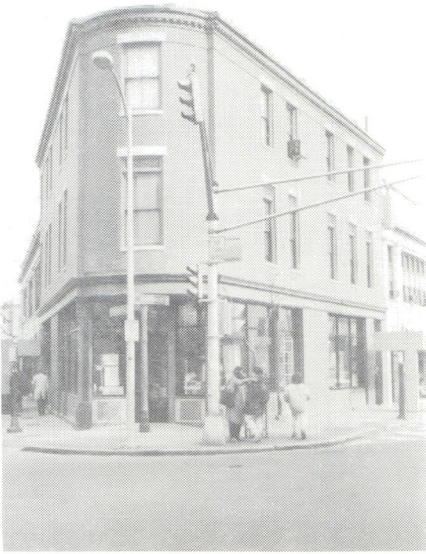
f) A 1775 structure which, though it once had a view of the Charles River, now looks out on railroad tracks and industry.
