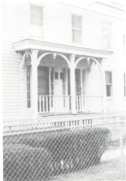
C12. Doubled-arched, double doorway
