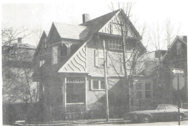
E22. Half timbers and fancy shingle work on a Queen Anne house
