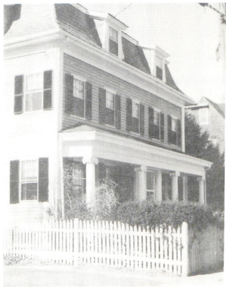
F4. Greek Revival house, with mansard roof
