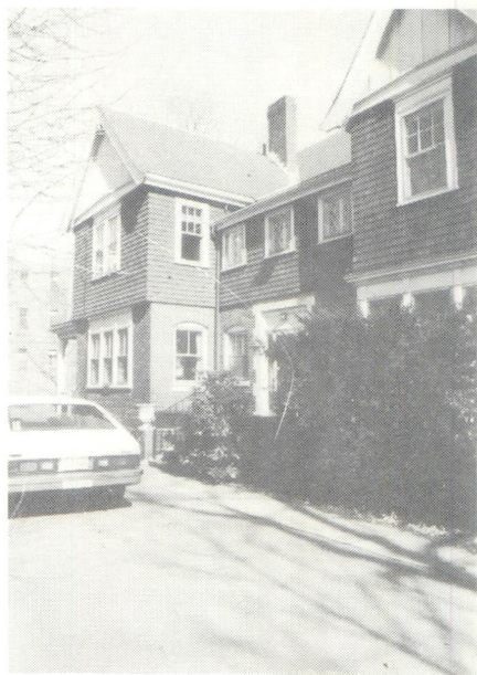
E21. Unusual side-entrance house
