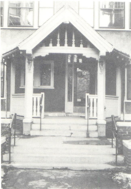
E13. Timber style entrance with balusters in the gable
