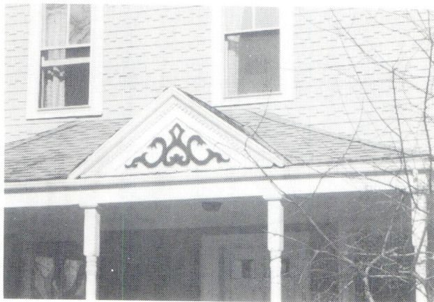
G23. Recently painted
