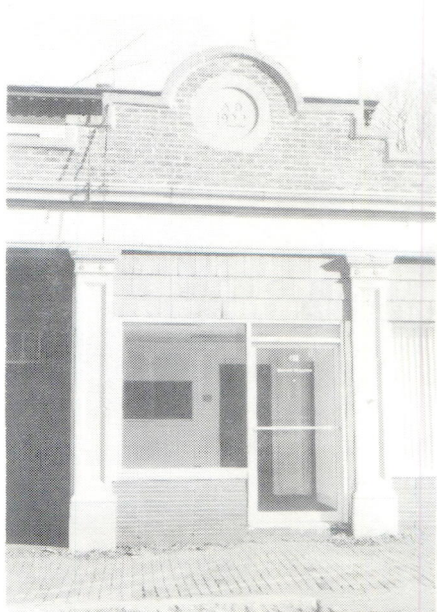
D21. Date in the roof line
