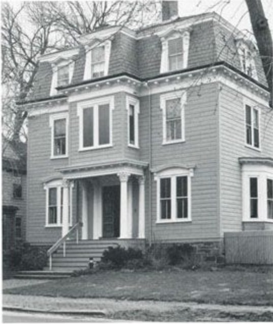
Figure 3. 77 LAKE VIEW AVENUE
