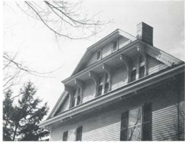
Figure 8. SOUTH GABLE OF 128 LAKE VIEW AVENUE
