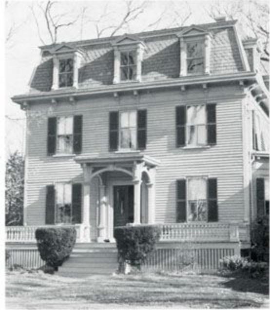
Figure 4. 87 LAKE VIEW AVENUE
