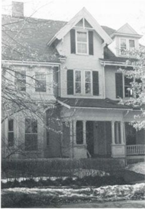
Figure 7. 128 LAKE VIEW AVENUE
