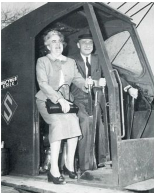
12. DEAN CRONKHITE AND PRESIDENT JORDAN BREAK GROUND FOR CRONKHITE GRADUATE CENTER. (Radcliffe College Archives)
