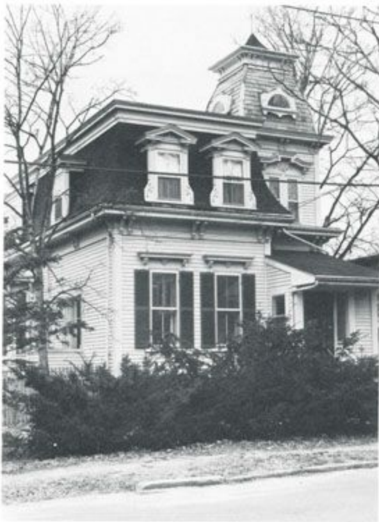
Figure 5. 94 LAKE VIEW AVENUE
