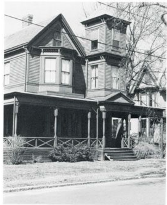
Figure 6. 78 LAKE VIEW AVENUE
