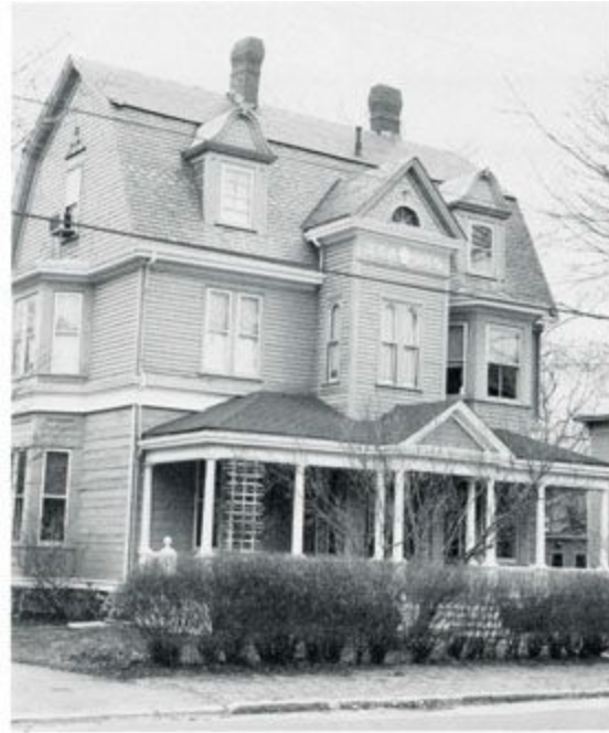
Figure 10. 58 LAKE VIEW AVENUE, AS REMODELED CA. 1894
